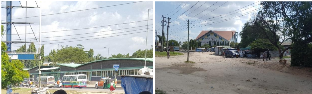
Figure 4: Power lines, Bus stop and business structures around the project site
